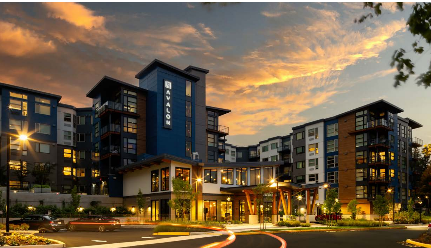
Campus de Avalon Redmond, Redmond, Washington
